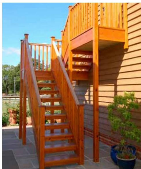
External staircase, property in Five Oaks
